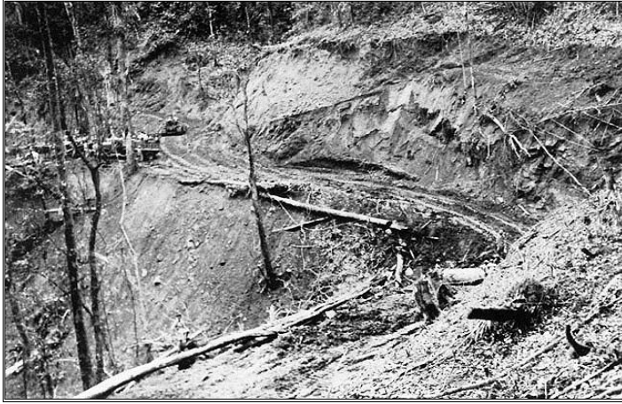
Army bulldozers constructing the Ledo Road cut a path through a hillside in the Indian jungle [http://www.ibiblio.org]
